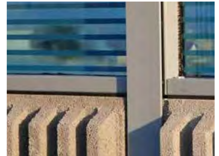
Integrated parapet and noise barrier system © Boscoltalia
