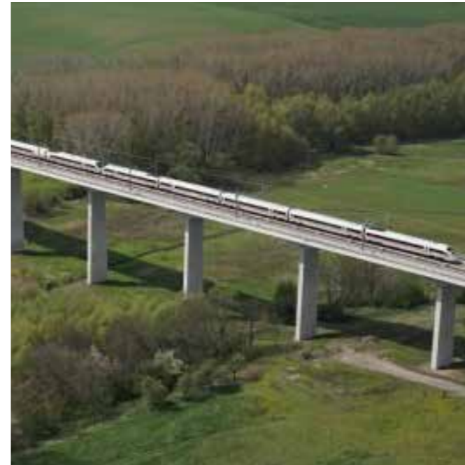
Scherkondetal railway viaduct near Weimar, Germany. Slender piers are elegant and piers at regular intervals allow reduced bridge deck. ©NormanHallermann
