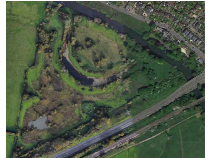
Attenuation pond and meander at Batheaston, River Avon. Ecological features include scrapes, wetland and scrub mosaic. The feature takes run off from the A4 Batheaston Bypass. ©2019 Google
