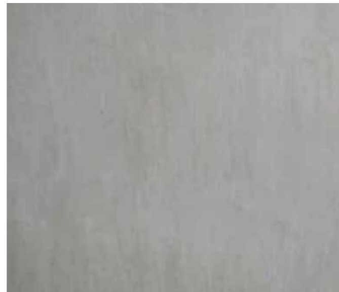
Well detailed, uniform concrete creates a high quality environment ©CRT
