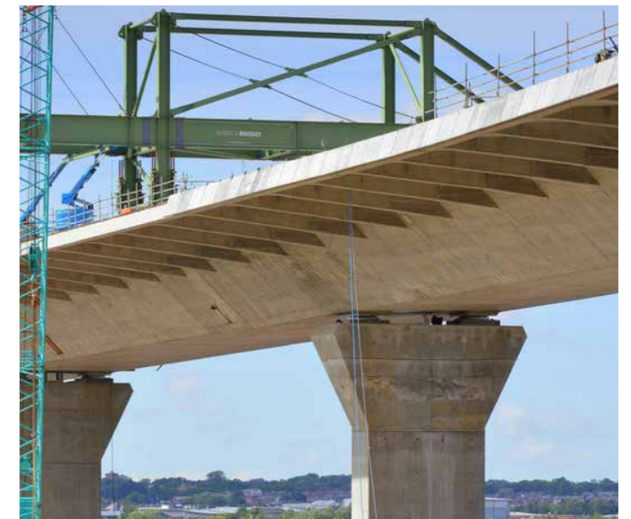
Ribbed cantilevered deck on the Mersey Gateway Bridge ©VincentPhillips
