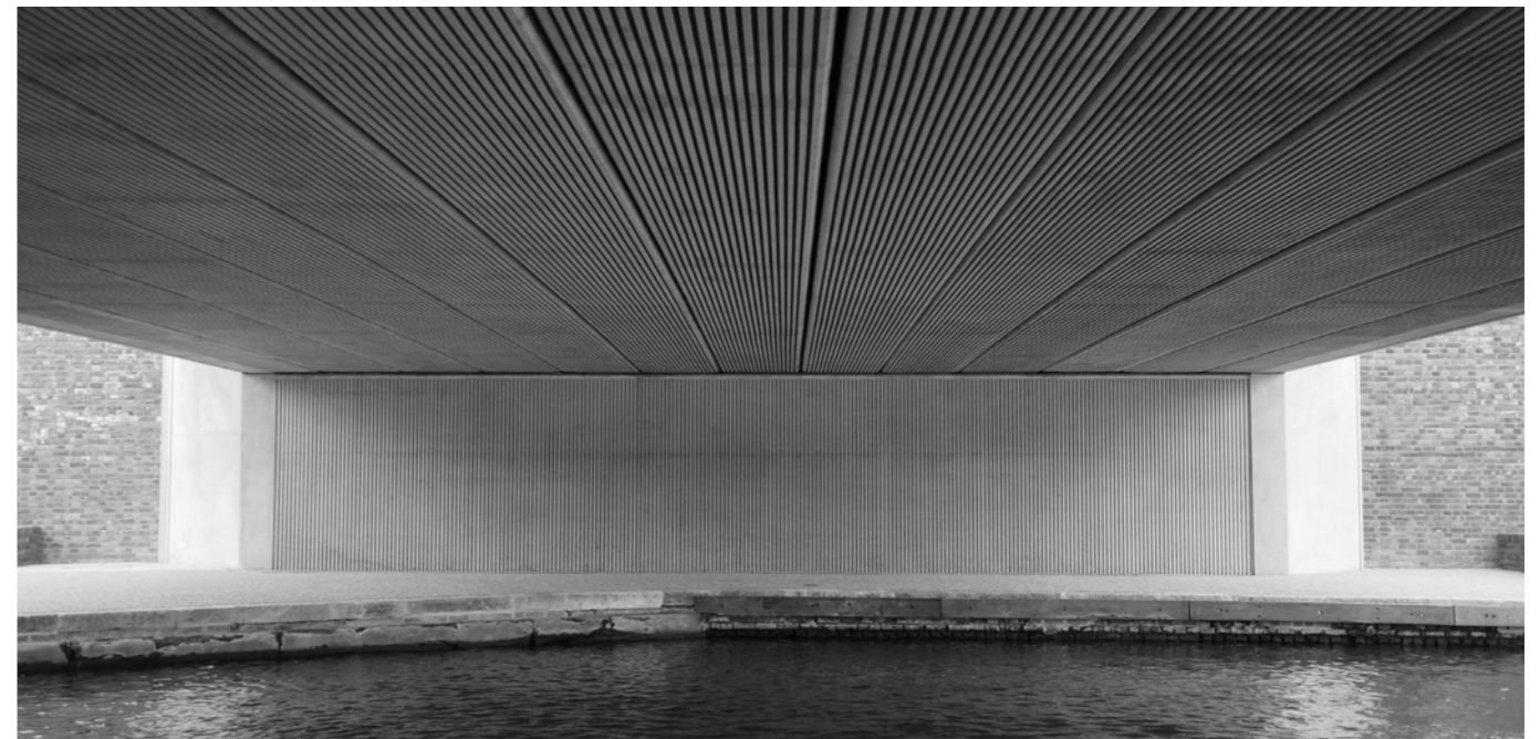
Ribbed bridge soffit, Kings Cross - texture and shadow visually reduce bulk of soffit ©KnightArchitects
