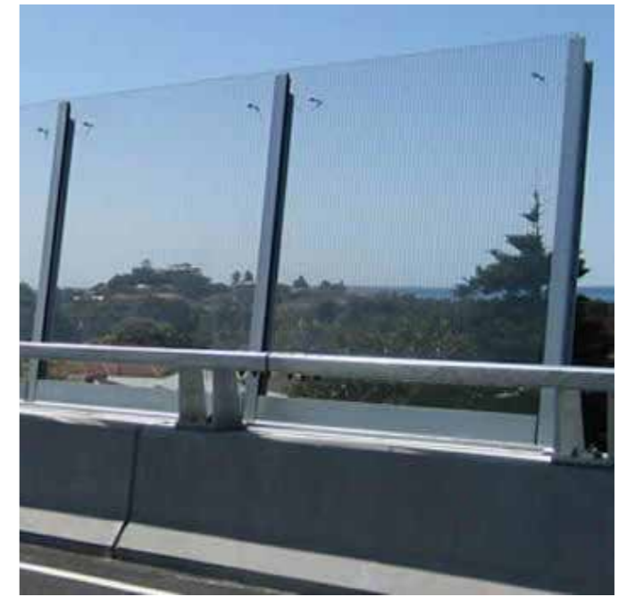
Use of transparent panels can reduce visual intrusion but can cause glare © Huanyu
