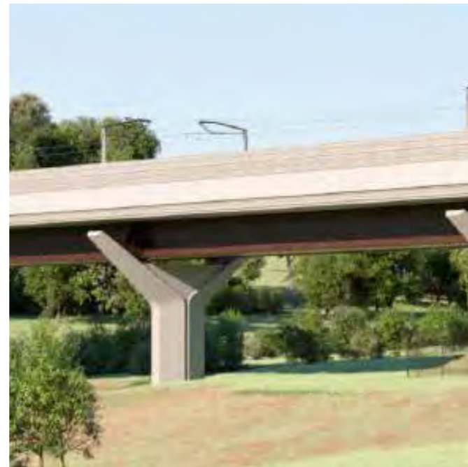
Exposed crossheads interrupt the viaduct soffit creating rhythm. Deck soffit colour and shadow reduces depth ©HS2
