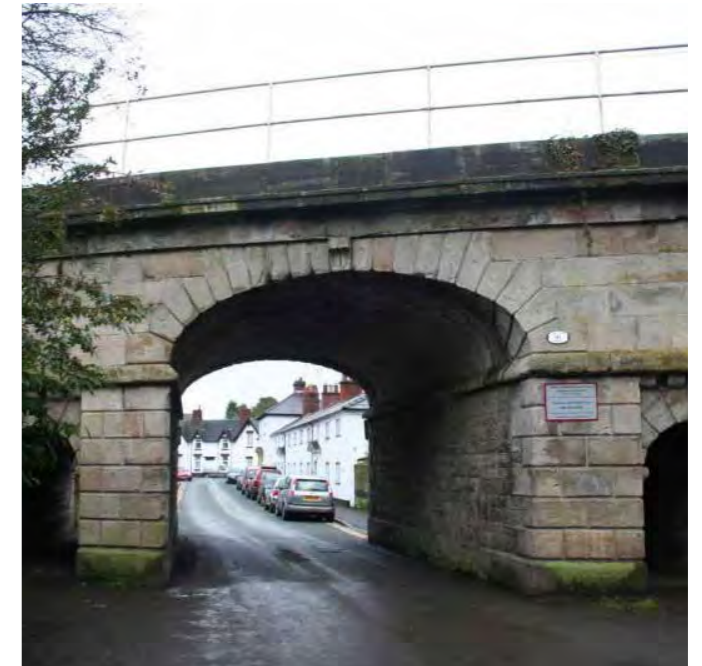
Railway bridge over Trent Lane creates a gateway into Great Haywood ©BritishListedBuildings
