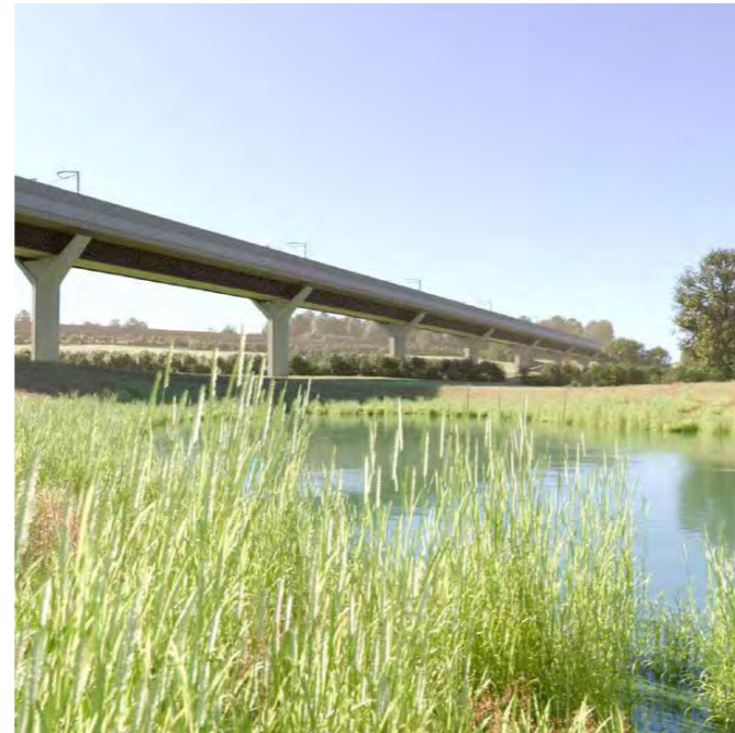
Chamfered parapet reducing bulk. Wendover ©HS2
