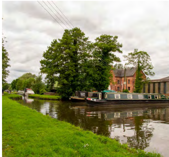
View along the Staffordshire and Worcestershire Canal with historic buildings associated with the canal
