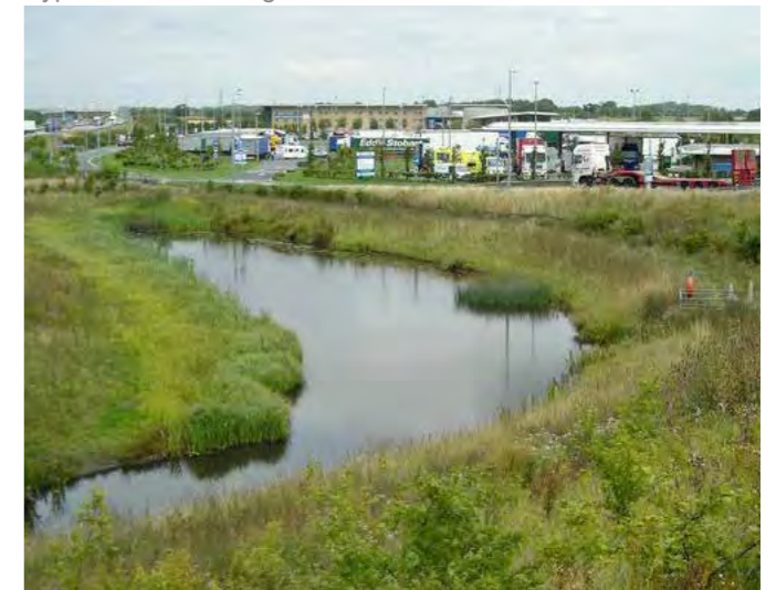
Well integrated attenuation pond, Wetherby Services ©AnthonyDixon
