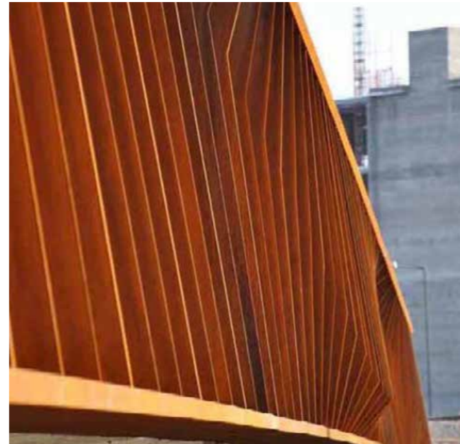
Weathering steel can form a positive elements to pedestrian environments ©CRT
