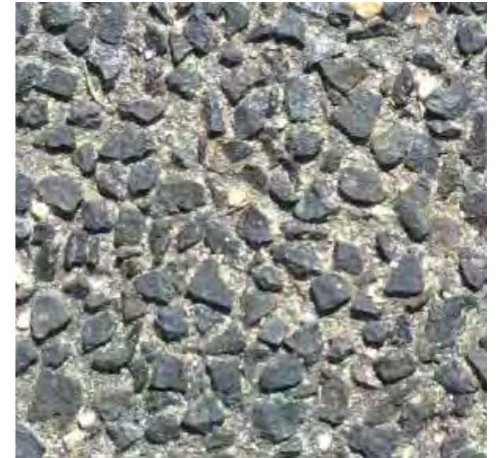
Exposed dark coloured exposed aggregate concrete
